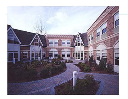
The new Assisted Living Facility featured two (2), 4 - story, 41,000-square-foot structures with 60-bed apartments / residence rooms, lounges, chapel, conference rooms, and a nurses' station with associated support spaces. The structural system includes concrete masonry bearing/shear walls, a large, steel-framed commons area, and several separate wood framed "cottage" apartments.
